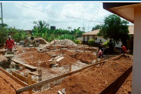
Construction site of AMR laboratory in Agroyesum, Ghana
